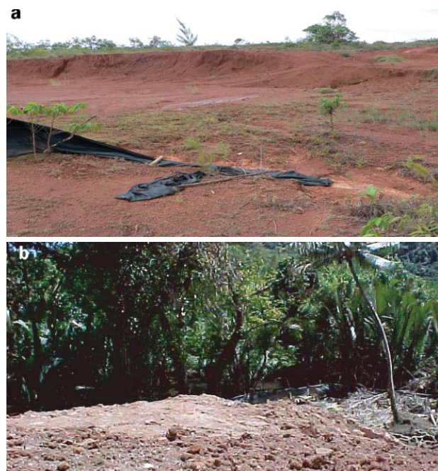
Figure 2. (a) An ineffective silt curtain. Developers usually obey rules requiring them to implement mitigation measures. These rules, however, usually do not state that the mitigation measures must be effective or that the developments and watershed alterations cannot result in the death of corals affected by discharges. Photograph: Eric Wolanski. (b) Mangrove forest in the Airai watershed, Palau, being filled for house sites. Silt screens in this area were ineffective and could not replace the buffering value of the mangroves and the associated bacterial and filter-feeding fauna. After data presentations and discussions among researchers, fishers, and local leaders, a moratorium was enacted to prevent any additional filling and destruction of this mangrove forest. Photograph: Robert H. Richmond.
